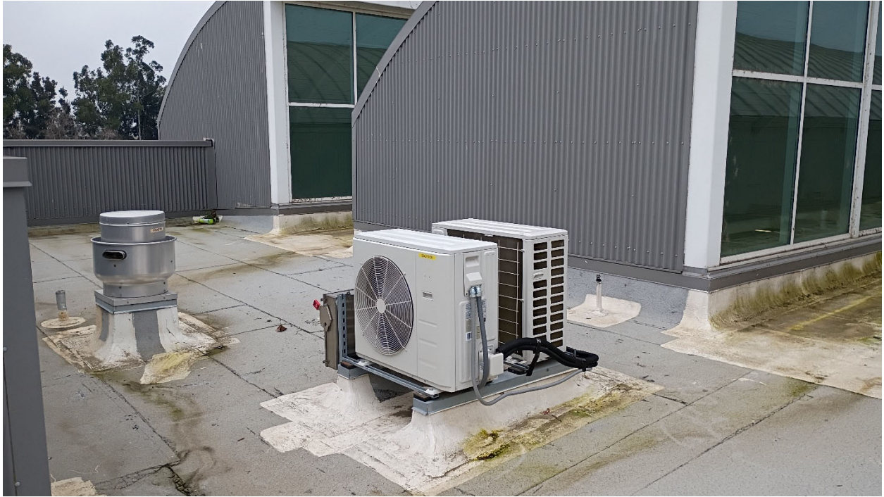
Pic – 5 East Side of Roof Looking Sout-West
