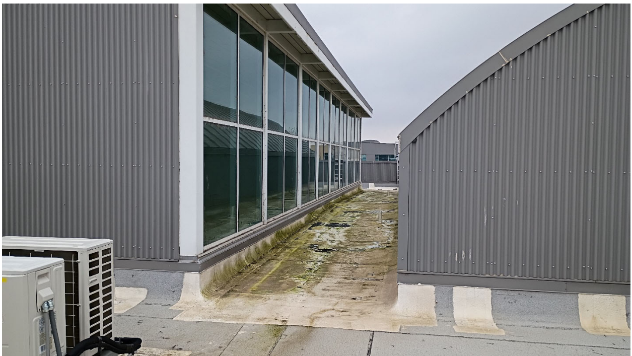
Pic – 4 Areas Between Curved Metal Roof
