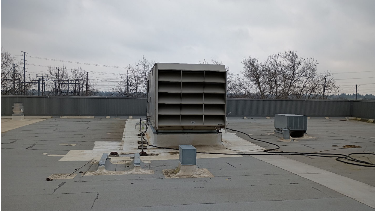
Pic – 3 Looking East to ACU15103
