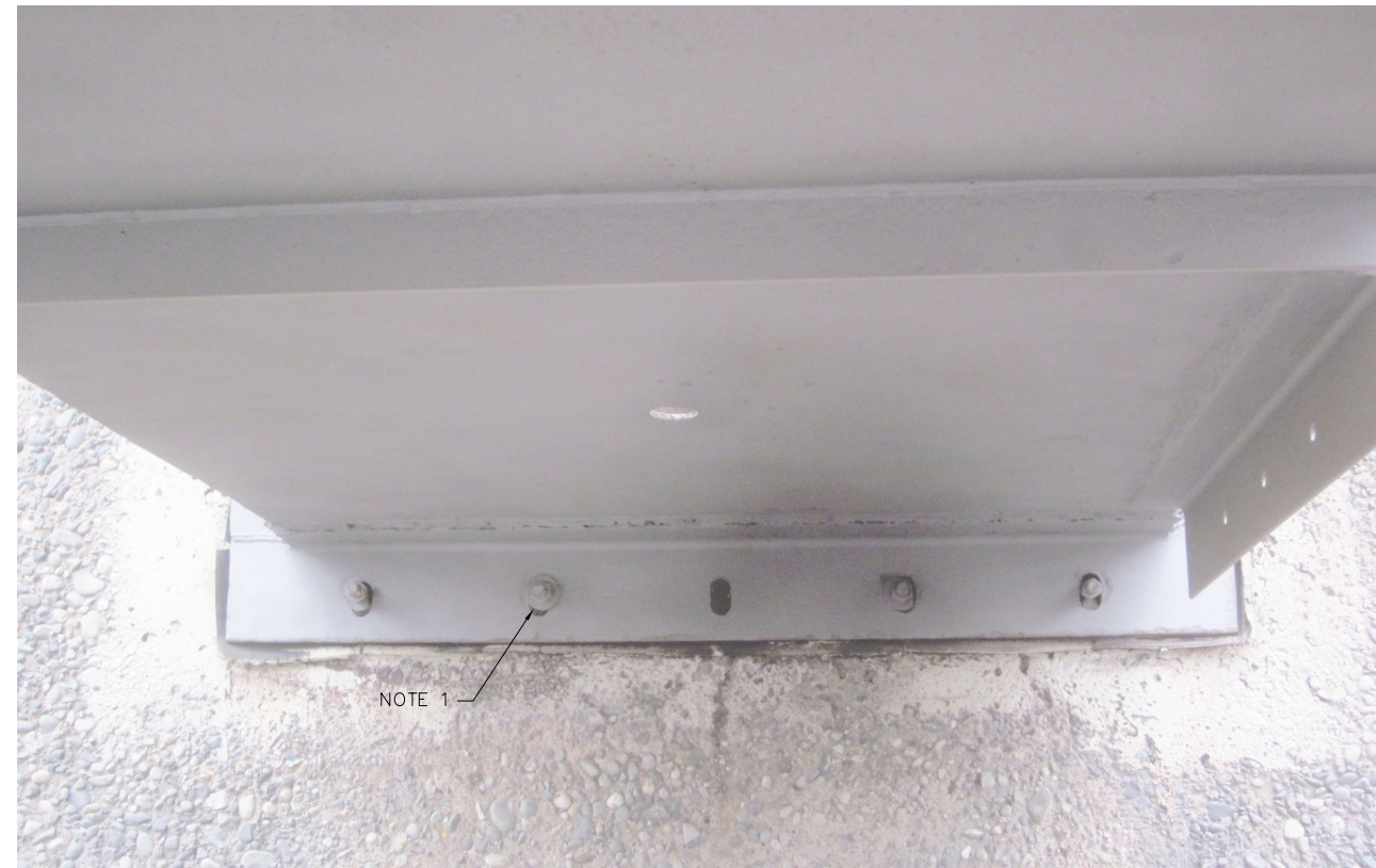
EXISTING LAUNDRER & CONCRETE WALL CONNECTION
